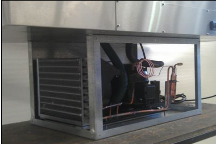
Condenser in Cradle attached under cabinet
